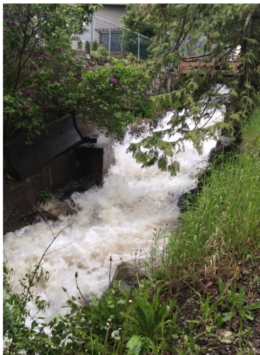
Figure 3-7. Anderson Creek between Gordon and Fell St. Note the make-shift mitigation works on the right (d/s looking) channel bank in the form of a jersey barrier. Photo: BGC, June 12, 2022.
