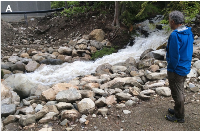
Figure 3-3. Anderson Creek near the fan apex. A) The left (west) lateral berm appeared to have been removed adjacent to the new water facility. Photo: BGC June 12, 2022. B) The left (west) lateral berm was replaced. Photo: Nelson, December 13, 2022.
