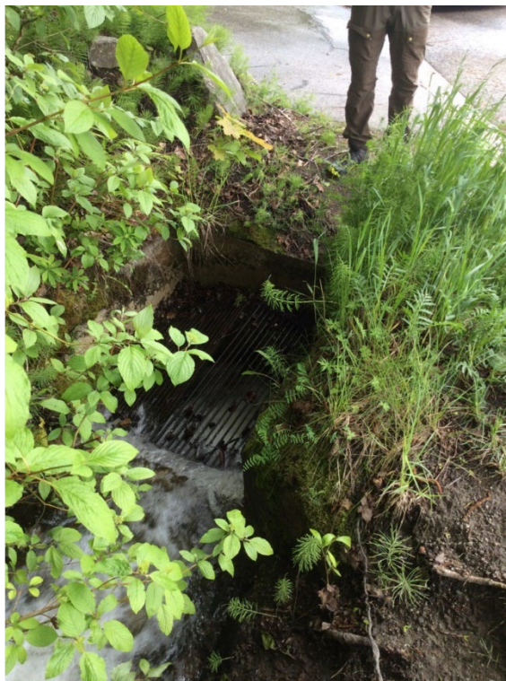
Figure 3-11. Culvert on Ward Creek at Fort Sheppard Drive. Photo: BGC, June 12, 2022.
