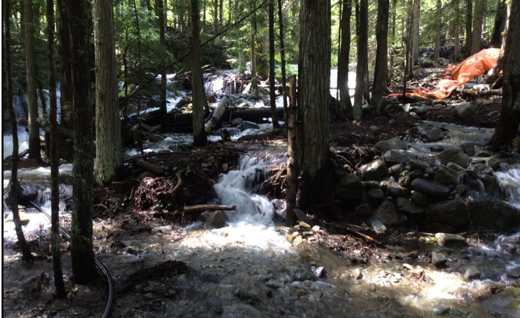
Figure 3-15. Giveout Creek through a poorly confined section of its fan. Numerous water intakes were noted with abundant pipes and other infrastructure in the flow path. Photo: BGC, June 12, 2022.
